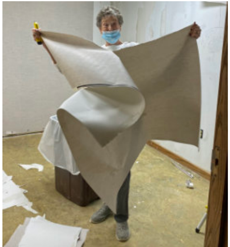
Judy Corwin, paper remover par excellence, virtually singlehandedly removed all the wallpaper in damaged areas.
