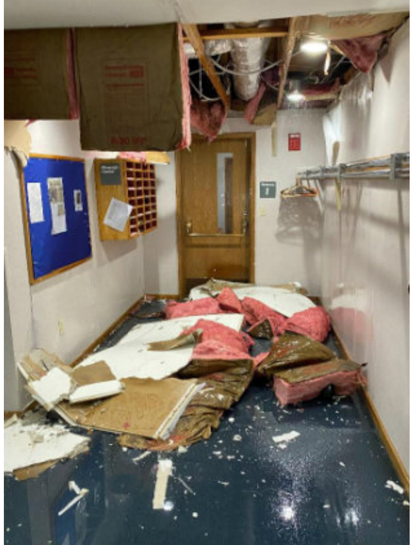
When ceiling water pipes burst, water and debris damage were everywhere in the east end of the Kirk complex. (Bob Morrow photo)
